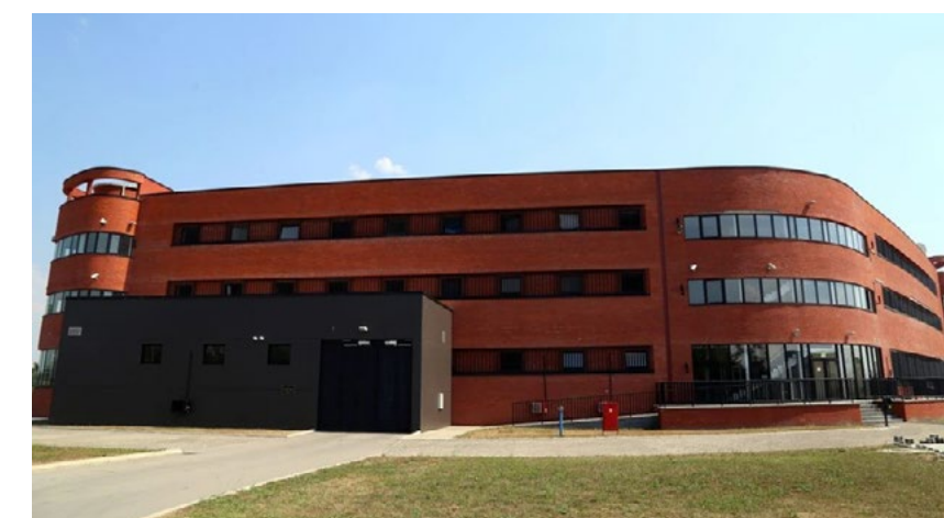
Exterior view of the high-security unit of the Penal-Correctional Institution Belgrade (Nova Skela), located in Padinska Skela, Belgrade
